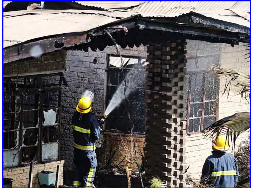
A firefighter douses the destroyed house following the tragic fire
