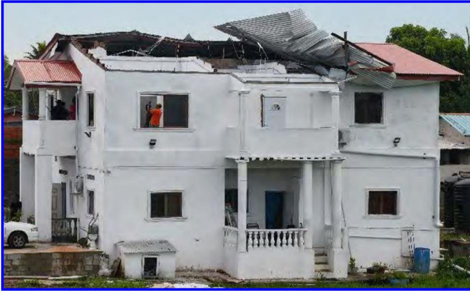
Wind-damaged roof of a house with missing sheets of galvanise
