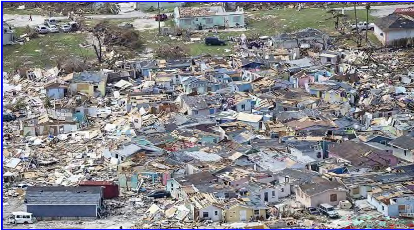
Extensive property damage in The Bahamas following the 2019 passage of Hurricane Dorian
