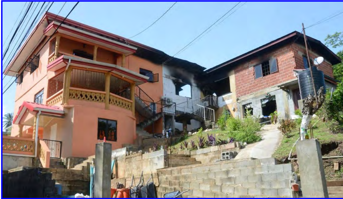
A firebombed Morvant house last week following ongoing gang warfare
