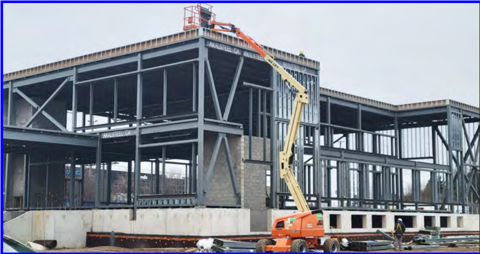
RKMCC's new building is well underway in Cambridge
