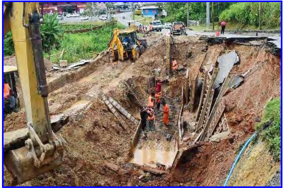
Repairs underway at the site of the extensive roadway slippage
