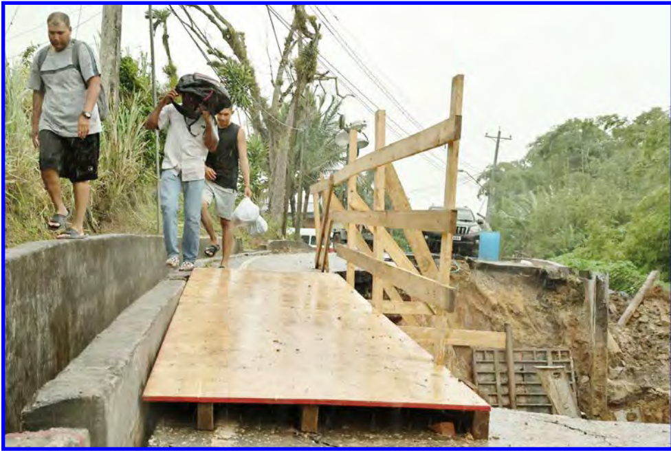
Residents cross a temporary bridge at the Brazil Arena Road
